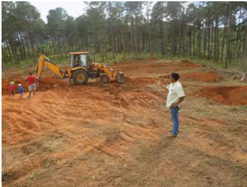
Ground levelling for RBI campus
