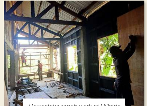
Downstairs repair work at Hillside
