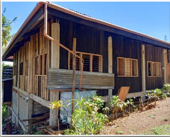
The Lacolac ministry center building repair...almost done.
