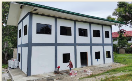
New church building under construction
